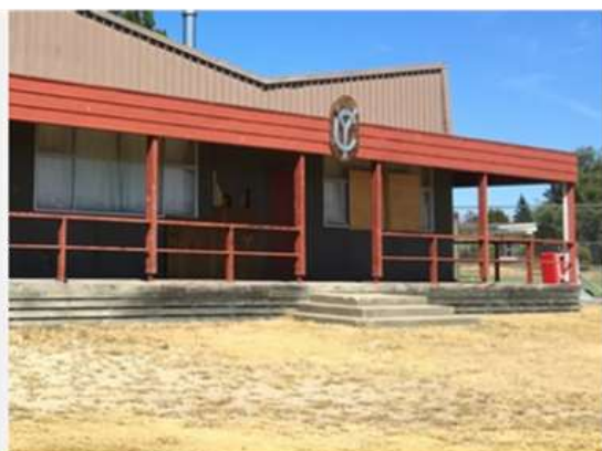
Photo 7. Main entrance stair without handrails
