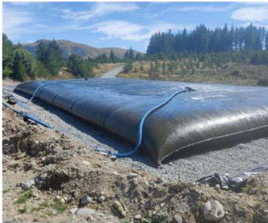
Heavy-duty bags being filled with sludge.
