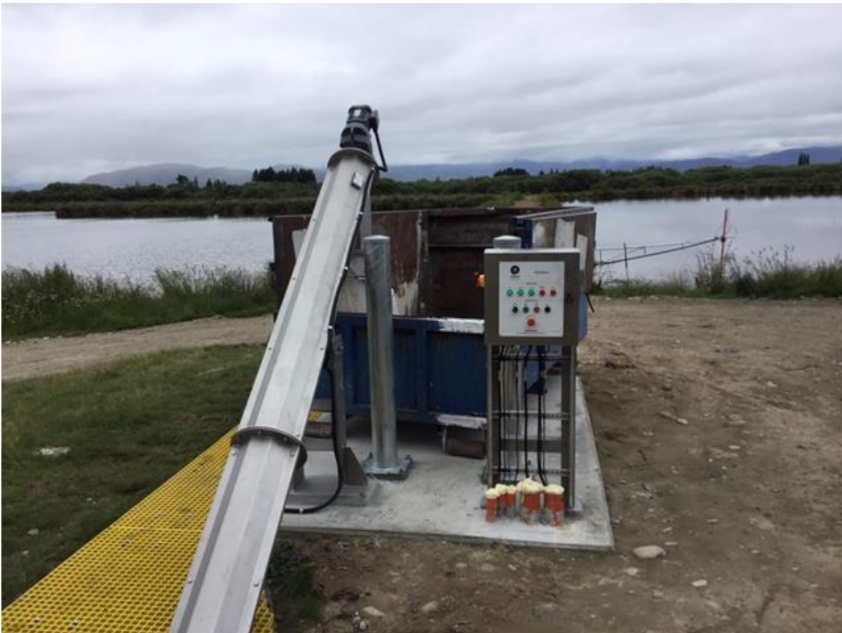
Mille Screen at Twizel Waste Water Treatment Plant.
