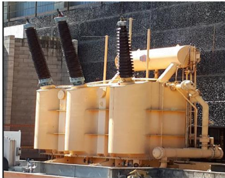
Image 4: The bushings or “insulators” on the transformers at the Ohau B powerstation
